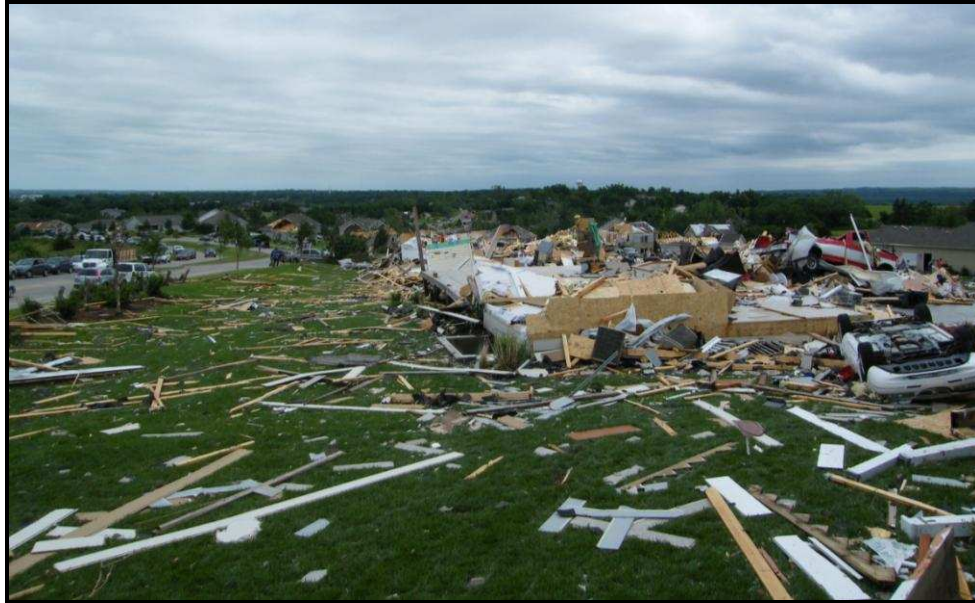
Figure 4.26: EF-4 damage in the Amherst residential area, Manhattan, KS (photo by author, taken with homeowner's permission, on 12 June 2008; the morning after the tornado).
